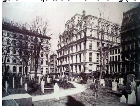
Figura 2 - Equitable Life Building (1870)
