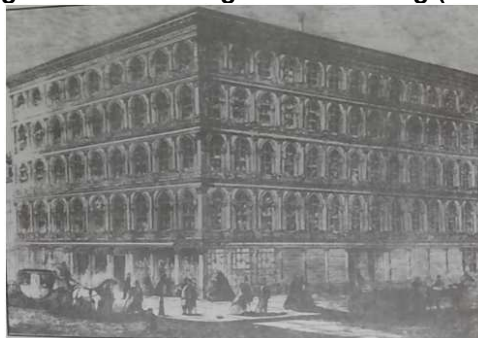
Figura 1 - E. V. Haughwout Building (1857)
